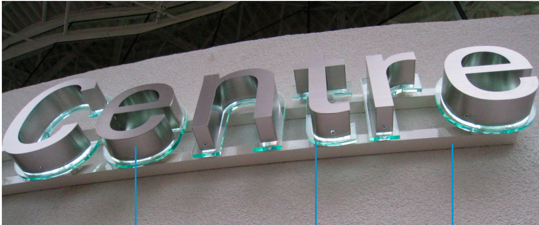
BUILT UP LETTERS WITH INTERNAL ILLUMINATION
